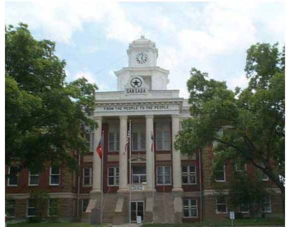
Credit: San Saba Chamber of Commerce
